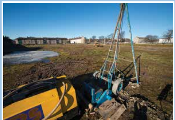
Summerhill Academy site Photo: Norman Adam, Aberdeen City Council
